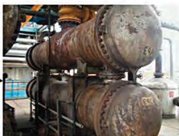
Design 2 Fouling factor from ‘design 1’ used in ‘design 2’, but actual fouling is worse!
