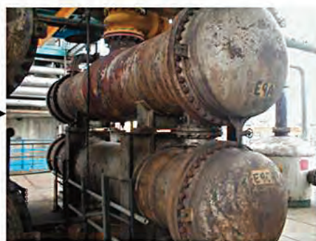
Design 3 Increased fouling factor from ‘design 2’ used in ‘design 3’. Actual fouling is even worse!!!
