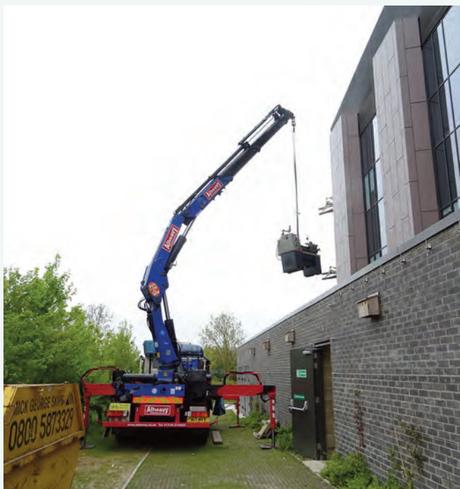
Crane lifting a lathe into the Mechanical Workshop in the new building
